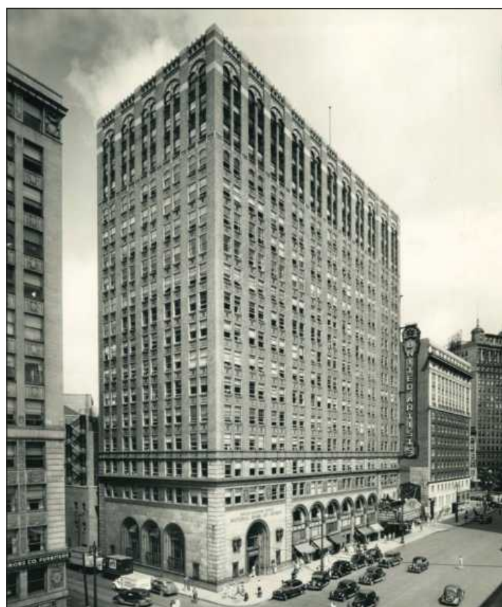
THE UNITED ARTISTS BUILDING in Detroit, in 1928. The 18-story building, mostly faced with orange brick, featured a 10-story blade sign signifying the building's theater. The sign was replaced in the 1950s.
